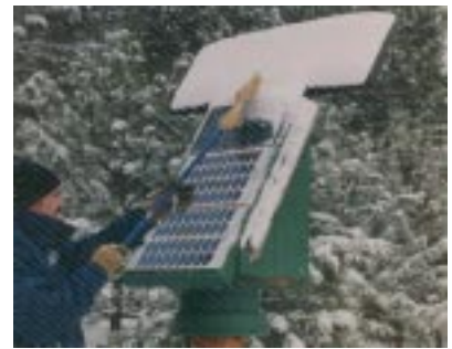
Our first solar panels mounted on a large tire rim providing an easy way to rotate the panels toward the sun.
