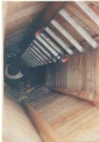
Walls of temporary wood framing holding the cement against the bank to provide the well casing.
