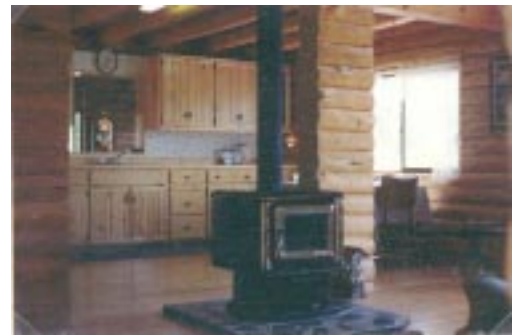
Cabinets are lodgepole pine. Stove hearth is made of white sand and masons cement using granite and marble stone set in a single iron framework. The floor is also lodgepole pine.
