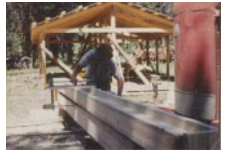
Fred using Alaska 3 chain saw mill to make a large upright support.
