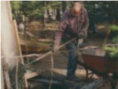
Fred pouring the cement down a wood slide lined with sheet metal, to form a casing inside the well.
