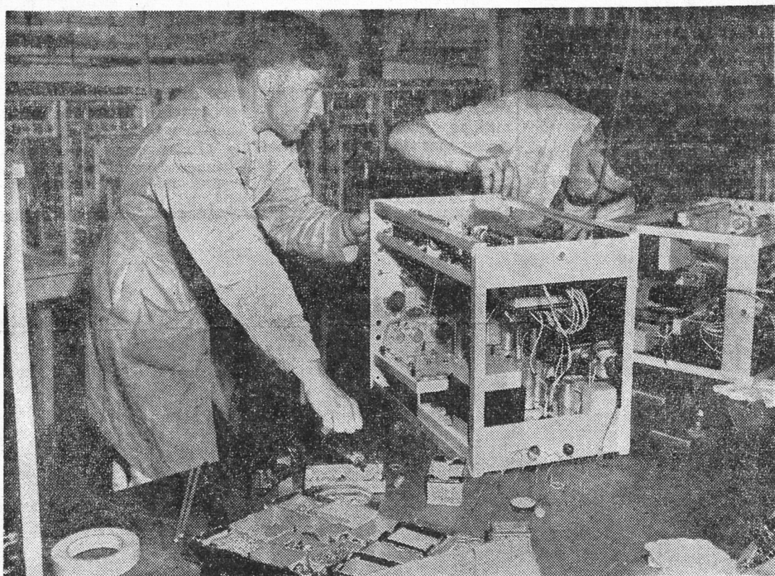
Ivan Arnold, left, 2741 S. E. 87th avenue, and R. J. Davis, 1704 S. E. Lexington street, assemble complex parts of a delicate electronic measuring device in Tektronics plant.
