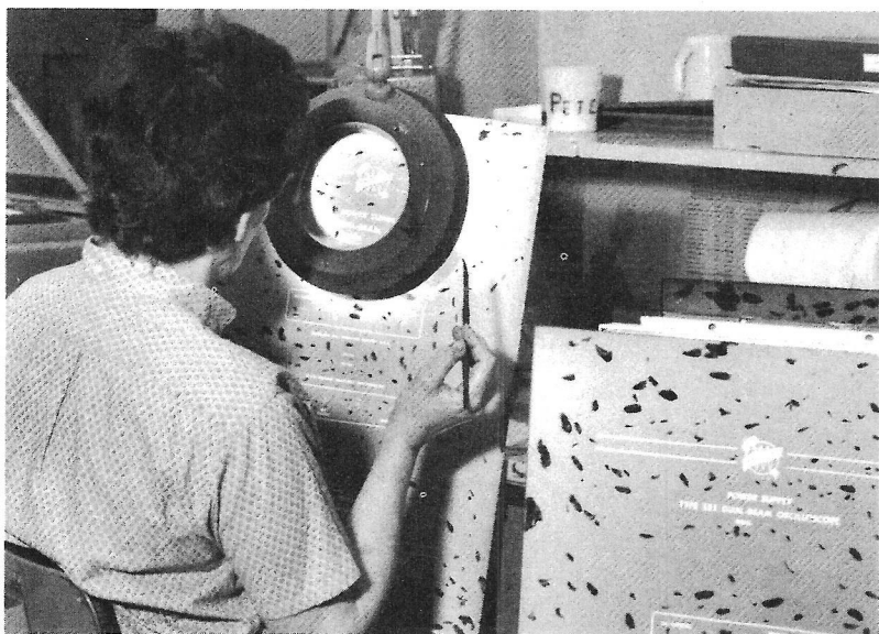
PANELS ARE SPOTTED to cover defects in the photo resist coating; from here they go to detail etching area (left). Control panel for automatic anodizing machine gets final check before production starts (right).
