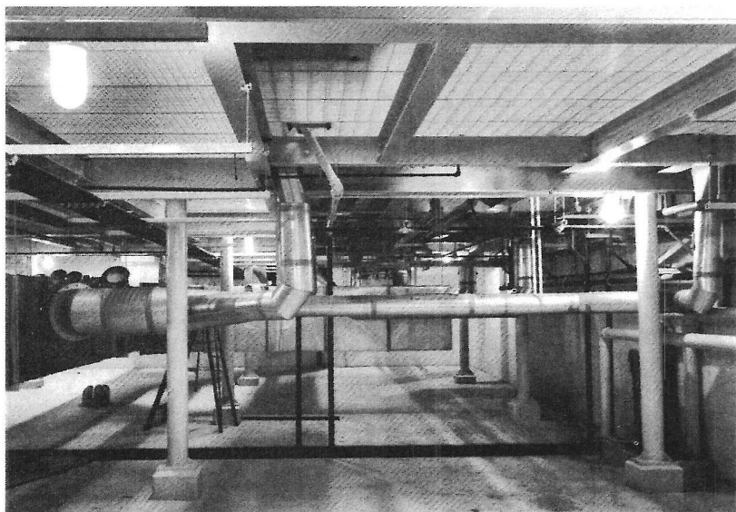
CHEMICAL PROCESSING FLOOR of new building holds all plating and anodizing tanks (upper left). Network of special resin-treated plumbing and ventilation pipes interlace under the chemical process area grids (lower left). Machine operator reproduces 24 panels at one time, using pantograph (right).
