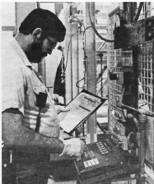
BOB KILLEN tells the computer about a batch of boards that he's starting down the plating line.
