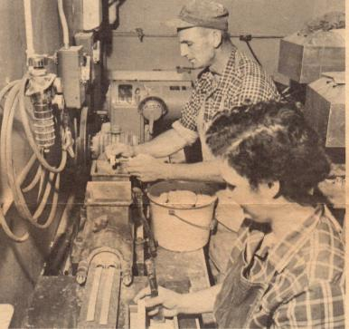
The ceramics department is expanding these days in other ways besides adding new girls. Our long hoped for extrusion machine finally arrived and is now installed and producing in the mold room in the quonset hut. Due to Jack Tate's ingenuity and the department's persistence the machine is producing at a good rate and improving daily, now that the usual wrinkles involving new machinery are ironed out.
