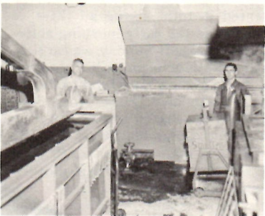
Roger Donato to the left handles the 'iron etch' and Dick Knight on the right chrome etches the panels. Note the hoist for sulfuric acid.
