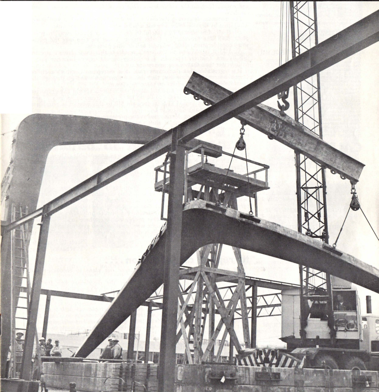
up go the concrete arches at our ceramics building
