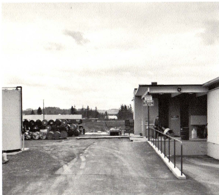
MAIN ENTRANCE (above) to Chemical Storage building includes driveway, loading dock (right), 3,500-gallon tank (left) and open storage area. The dispensing room (below) has air vents near ceiling for adequate ventilation. A lanyard is strung along room (see arrow) which employees may pull in an emergency to obtain outside help.
