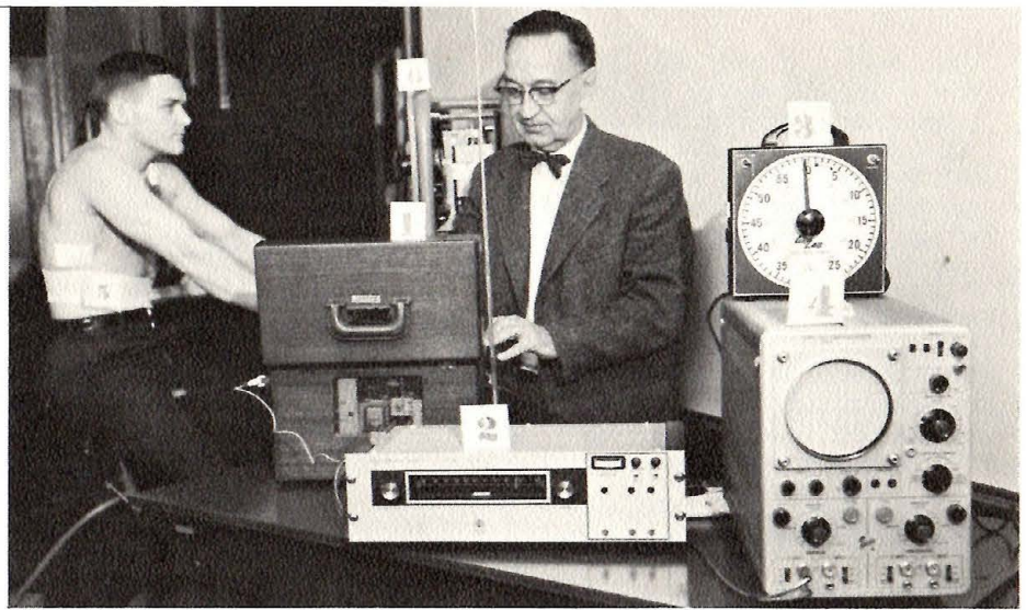
Dr. Herman Gawer (right) of OSU demonstrates telemetry system used to test athletes' heart action under measured amount of strain. Type 503 is used in project which may extend the uses of an electrocardiogram to persons engaged in strenuous activities.
