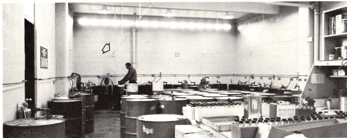
MAIN ENTRANCE (above) to Chemical Storage building includes driveway, loading dock (right), 3,500-gallon tank (left) and open storage area. The dispensing room (below) has air vents near ceiling for adequate ventilation. A lanyard is strung along room (see arrow) which employees may pull in an emergency to obtain outside help.
