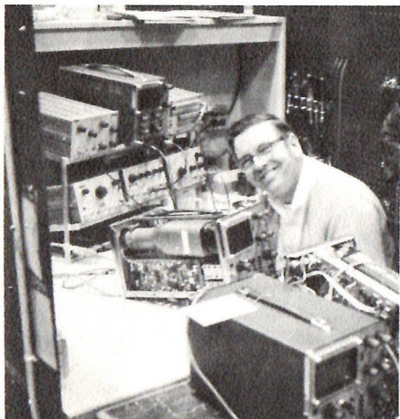
TOM HERD tests first Telequipment D54 instrument to be assembled at Tek Beaverton. The D54 is a 10 MHz oscilloscope.
