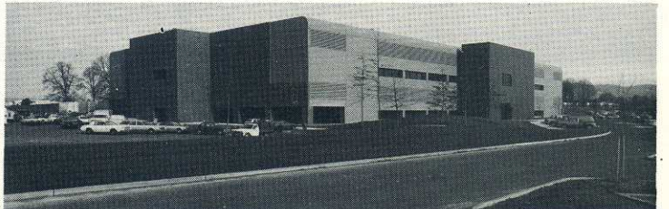
Building 59 - The Microelectronics Design and Manufacturing Centre at Tektronix Industrial Park in Beaverton, Oregon.
