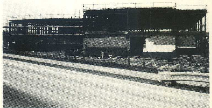
Two views of the new building at Marlow.
