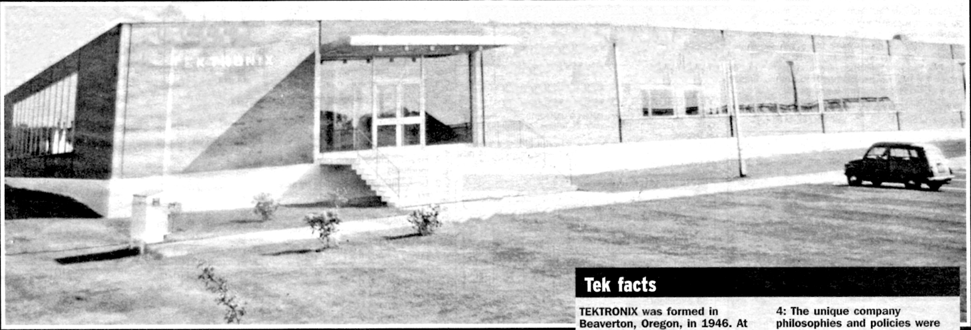
The purpose-built and state-of-the-art premises at La Villiaze, to which the company soon moved and which is now occupied by Specsavers. (1195096)
