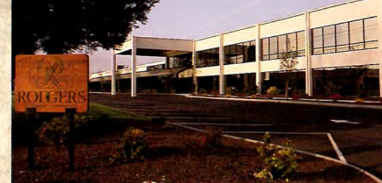
Rodgers international sales and administrative offices and manufacturing facility in Hillsboro, Oregon.
