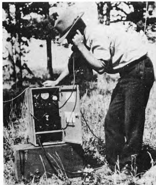
Figure 72. Type TH/TL in semiportable configuration for field use. See figure 97. (NA:95G-316855)
