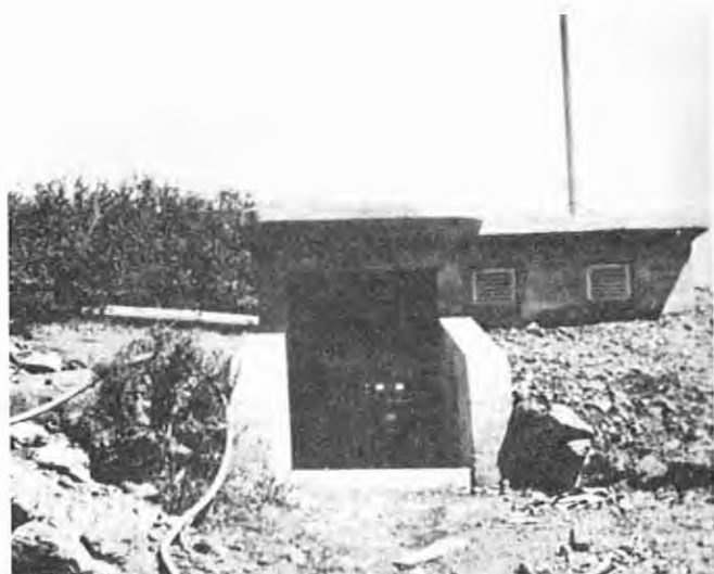
Figure 77. The RRS (Radio Relay Station) installation atop Mt. Diablo, Calif., first field setup of the Forest Service, July 1941. It allowed the nearby Regional headquarters in San Francisco to establish point-to-point communication with any outlying vhf radio within visible range of the repeater. Esthetics required the RRS to be placed in a plain building that minimized environmental impact. (Forest Service photo, History Section)
