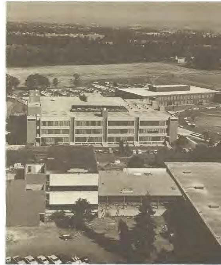
FOREGROUND: New component-manufacturing building.
