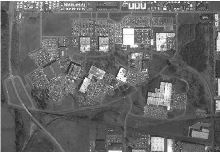
1976: 16 (Mech Products), 48 (Electron Devices), 58 (Gen'l Purpose), 55 (Operations), Murray Rd is complete (Left Side)
