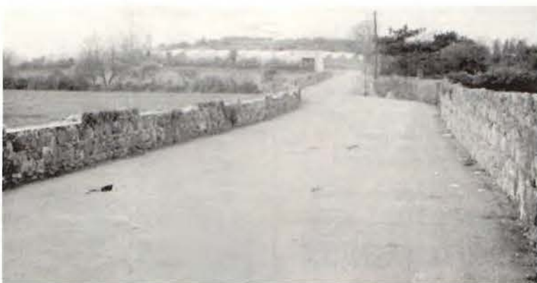
Approach to the plant site at Guernsey.
